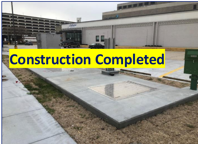
Houma & W. Esplanade Lift Station Upgrade Project $1.5 Million)
