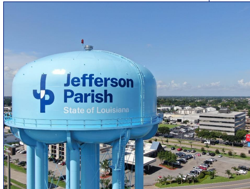
I-10 / Causeway Blvd. Water Tower
